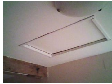
Heat leaks around hatch.
