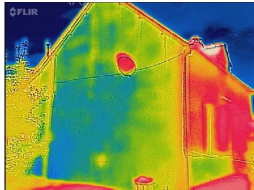
Note contrast with east-facing traditional wall.
