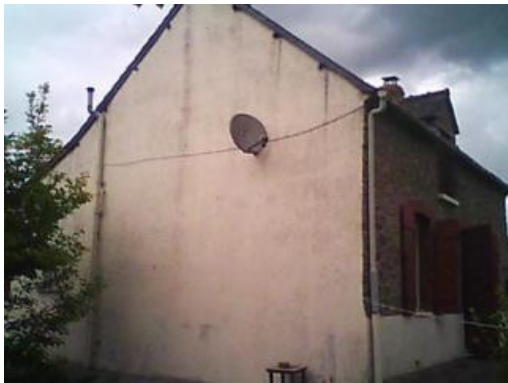
South-facing wall (rendered).
