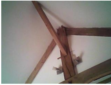
Missing insulation to roof void and pitch.
