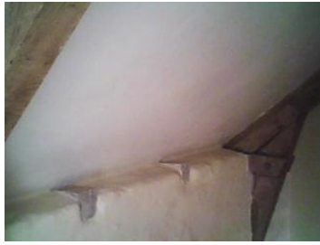
Missing insulation to roof void and pitch.
